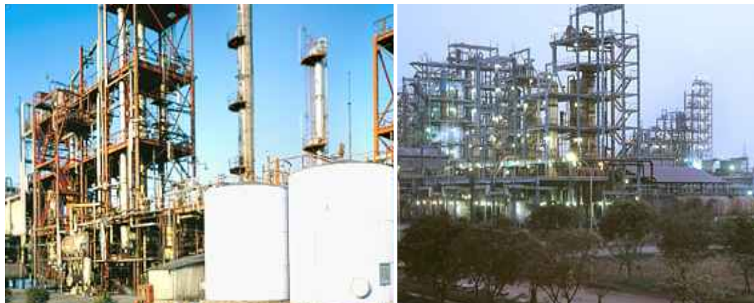
Jubilant's manufacturing facilities at Gajroula and Nira.
