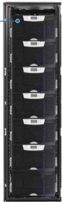
Redundant N+1 configuration: Six 12 kW UPS modules share the load equally. If a UPS module is removed from service, the remaining modules seamlessly support the load without interruption.
